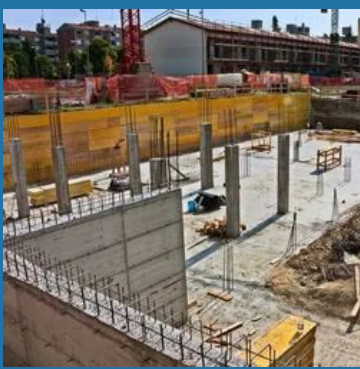
Commercial Buildings Construction
