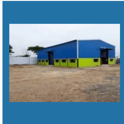
Commercial Building Construction Services
