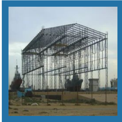
MS Shed Fabrication
