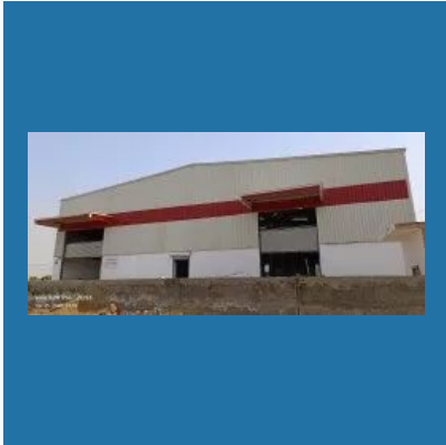
Industrial Shed Construction
