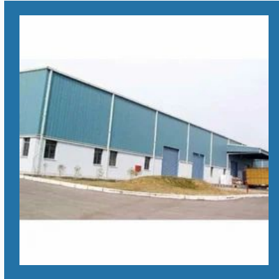
Fabricated Industrial Shed
