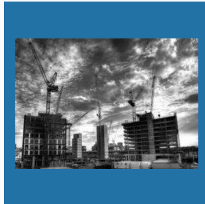
Commercial Construction Projects
