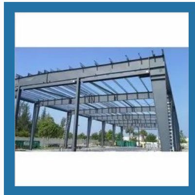
Fabricated Building Construction
