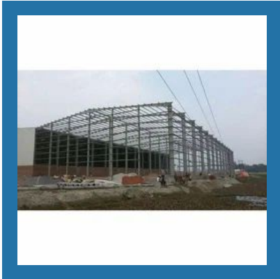
Warehouse Shed Structure
