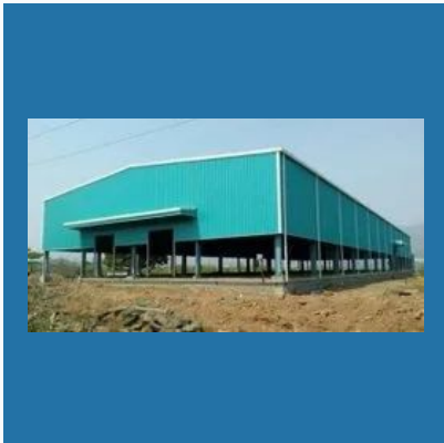
Fabricated Tin Shed
